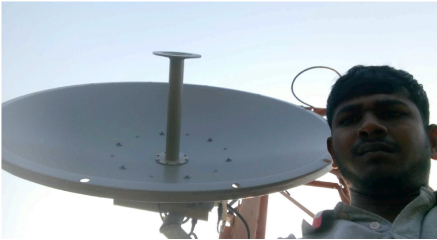
Technician installing the link
