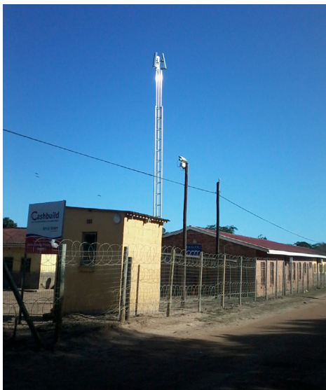
ePMP Access Point tower at school
