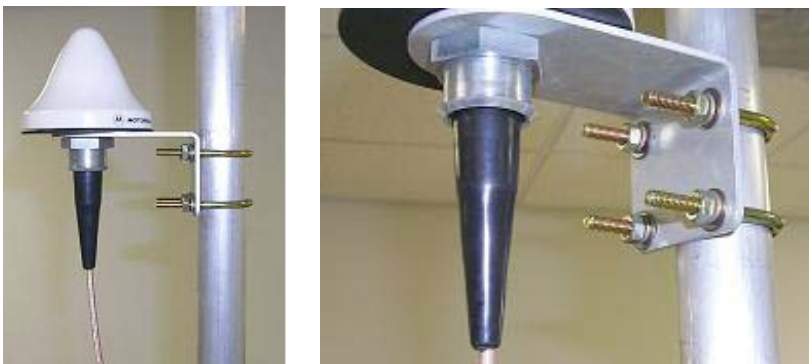
Figure 29 Detail of GPS antenna mounting
