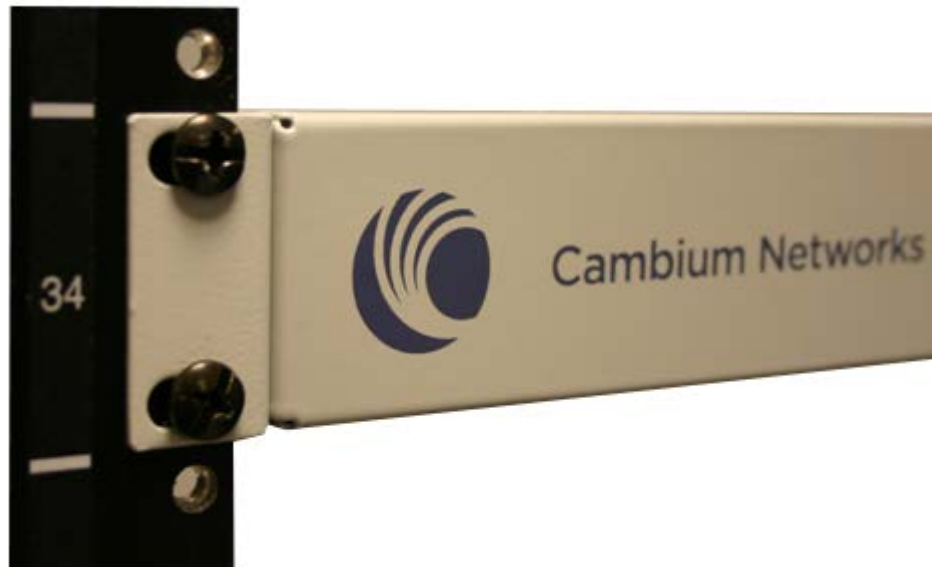
Figure 39 Rackmount CMM4 rack screws
