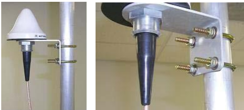
Figure 55 Detail of GPS antenna mounting
