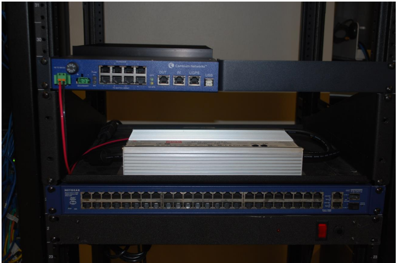
Figure 23 600 Watt Power Supply Installation
