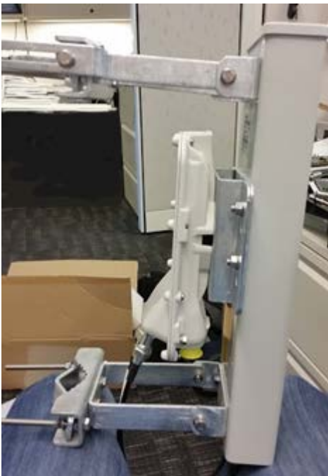
Figure 95 Completed AP and antenna assembly
