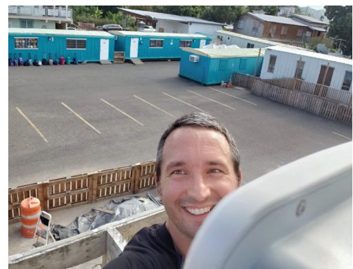
Charlie Galik installs a cnPilot™ e700
