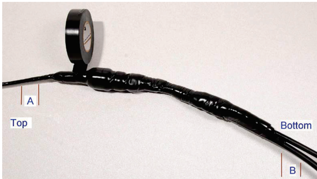
Figure 113 Wrapping PVC tape around the GPS adapter cable joint
