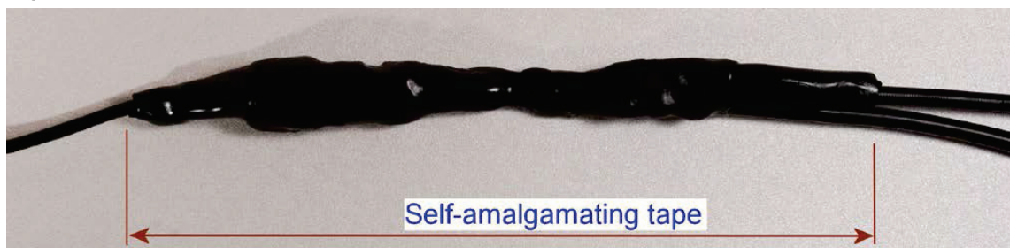
Figure 112 Wrapping self-amalgamating tape around the GPS adapter cable joint
