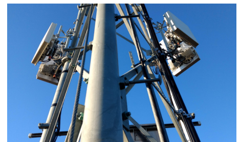
Narrow beams created in MU-MIMO mode increase coverage and throughput while reducing the system’s interference.
