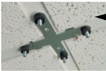
T-Bar Bracket (with spacers installed)
