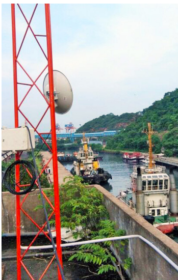
eMP solutions brought field-proven reliability, GPS-sync-enabled scalability and high-quality performance to the port yard and construction roads.
