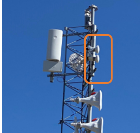
A small form factor dual-horn antenna uses less tower space
