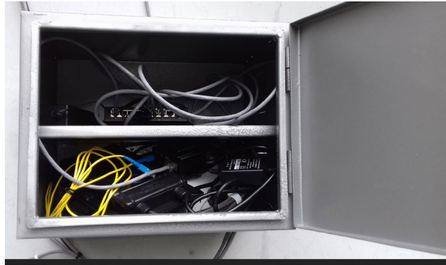
Figure 2-9 Outdoor Power Supply installation
